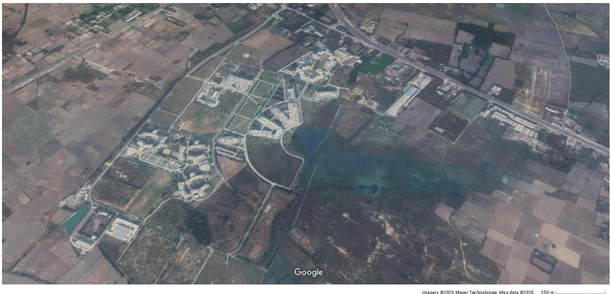
Above: ‘ Space before and after the establishment of Shiv Nadar University’
